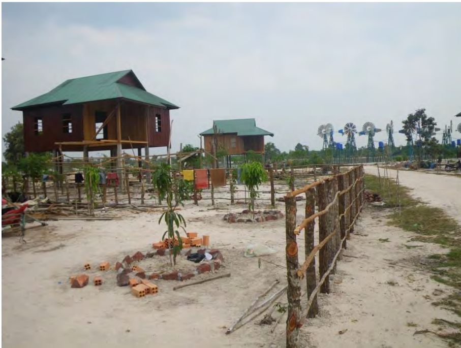
Fig. 2: Houses under construction in Run Ta-Ek (2011).
