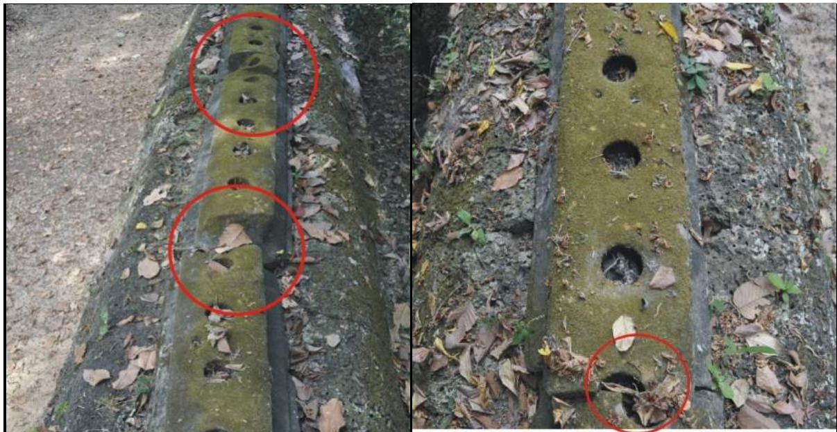
Figure 6.8 – Coping stones on the West wall - Note the breaks and broken ends.
