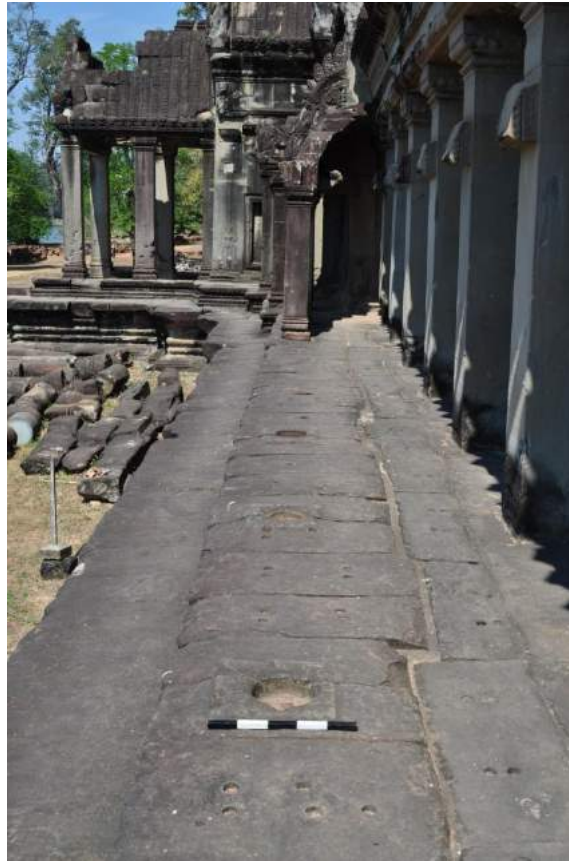
Figure 6.2 - West gopura, exterior, facing South – Note the postholes for the verandah columns (foreground), the sheared cross beams of the verandah (right), the missing stones of the porch roof (background, left) and the original verandah column and corbel vaulted roof in situ (background, centre)
