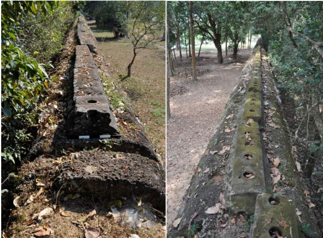
Figure 6.5 - Coping stones along the top of the West wall – Note the elongated shape.
