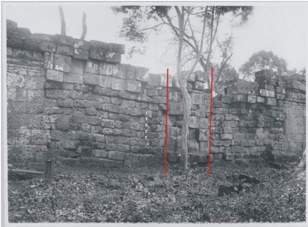
Figure 5.26 – South wall, West gateway, showing the pattern of laterite and sandstone components (EFEO archives)
