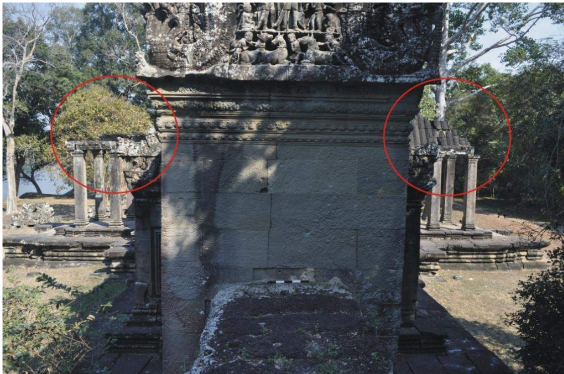
Figure 6.3 - North gopura, facing East - Note the missing stone pieces from the porch roofs and the architraves.
