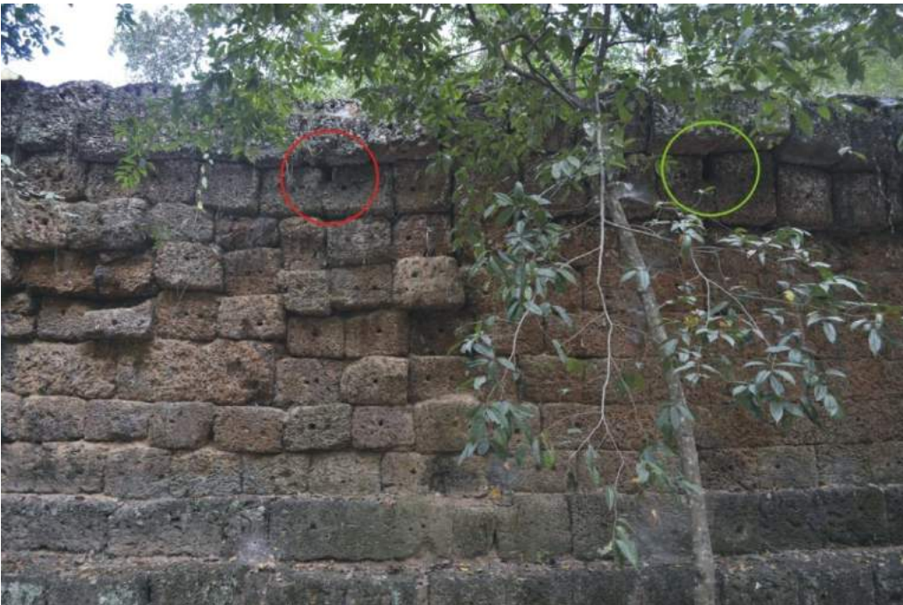
Figure 5.29 - Horizontal postholes in the original wall (green) and the later modifications (red) –North wall, East gateway (above), East wall, North gateway (below)
