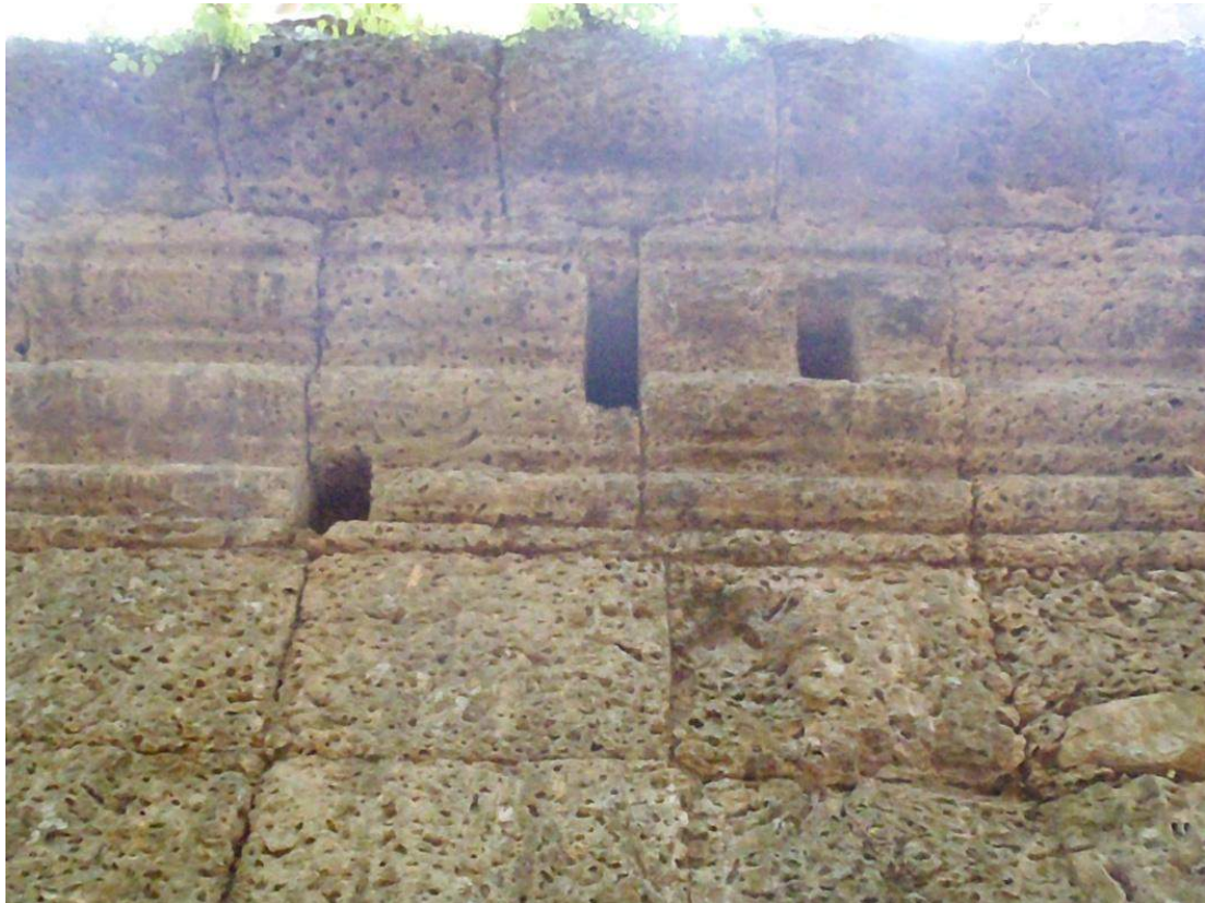
Figure 5.9 - A cluster of postholes: South wall, West side, near the South gopura.
