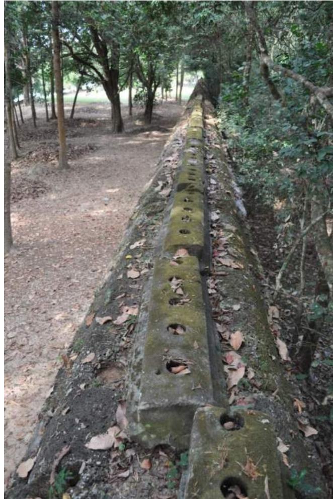
Figure 4.11 - Sandstone coping stone with postholes for finials, West wall facing North.
