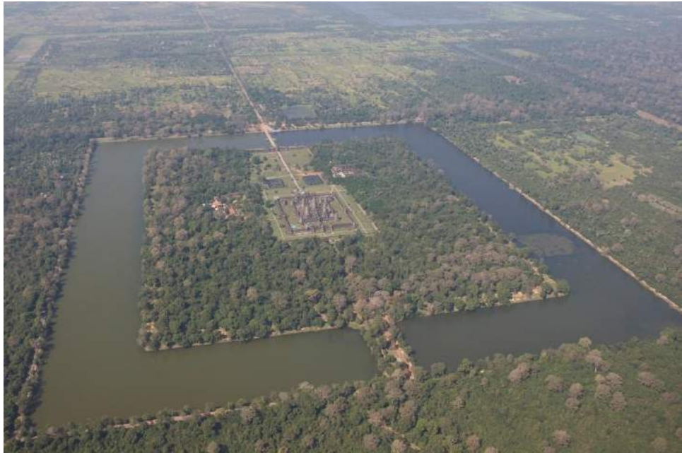
Figure 1.1 Angkor Wat, facing West (Dago 2010)
