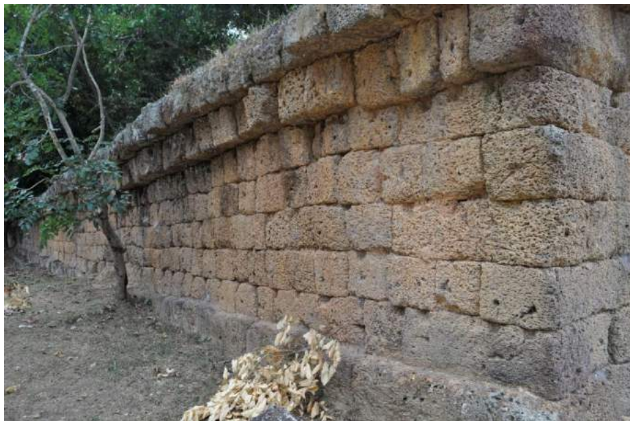
Figure 4.7 – Indentations, Northeast corner, exterior – Note their presence at all heights of the wall
