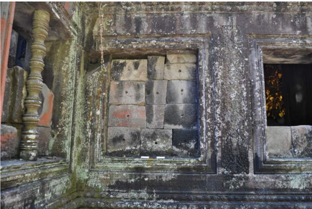
Figure 4.31 - The difference in block work between a false window (above) and real window with blocked up infill (below); South gopura, interior.
