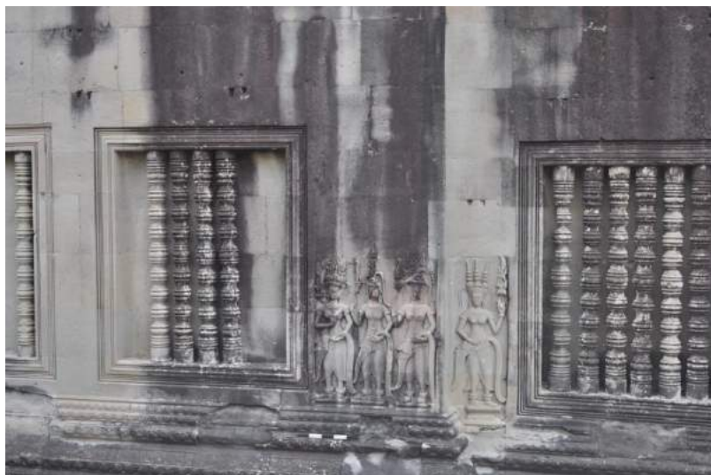
Figure 3.4 Real (above) and false (below) balustered windows in the inside wall of the second gallery
