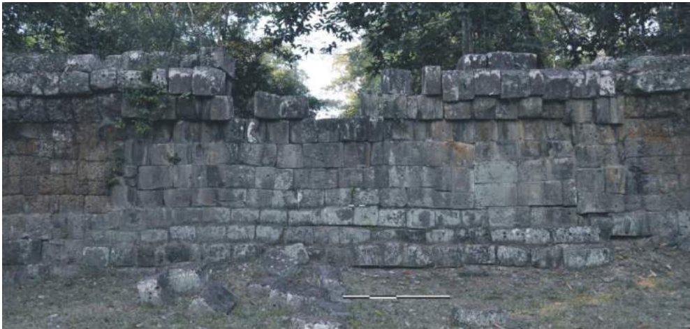
Figure 4.18 - Photo and masonry pattern of the South gateway on the East wall – laterite (white), termite mound (beige)
