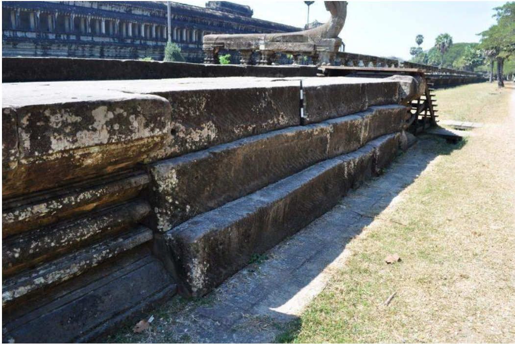
Figure 4.21 - Central Northern staircase between the ground level (right) and intermediate level (left)
