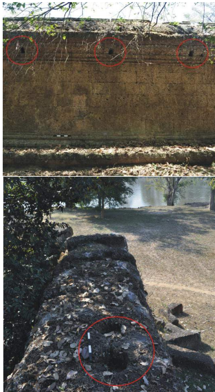
Figure 1.5 – Postholes in the fourth enclosure wall: horizontal on the inside face (above) and vertical on top (below)
