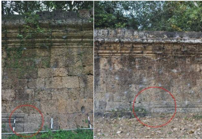
Figure 4.27 - Changes in surface finish detail in the South wall, West sector, exterior, near the West gateway –West of the gateway (left) and East of the gateway (right)
