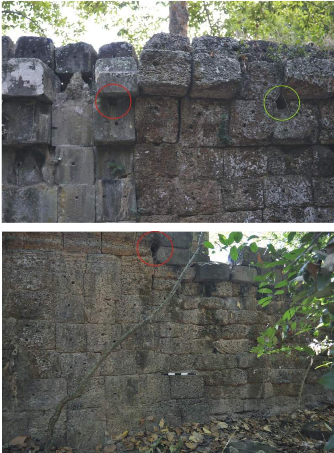
Figure 5.30 – Horizontal postholes in the original wall (green) and the later modifications (red) – South wall, East gateway (above), South wall, West gateway (below)
