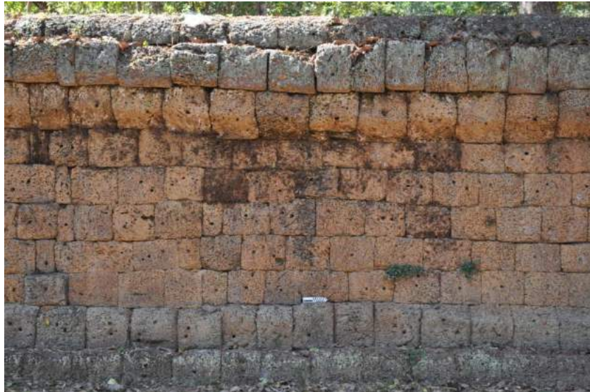
Figure 4.5 - Manoeuvring holes in the exposed face
