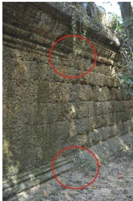
Figure 4.28 - Changes in surface finishing detail in the North wall, West sector, interior, near the West gateway (to the right of frame)
