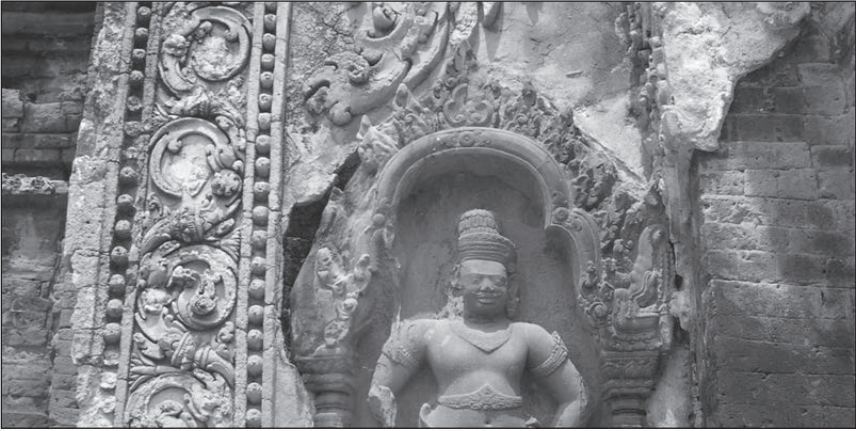
Figure 13.3 Stucco rendering laid over brickwork amidst a sandstone representation of a dvarapāla at Preah Kō.
