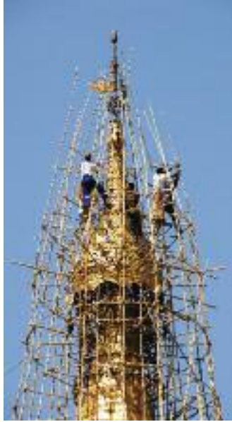
Workers stabilizing the metal hti capping the Alodawpyi temple.
