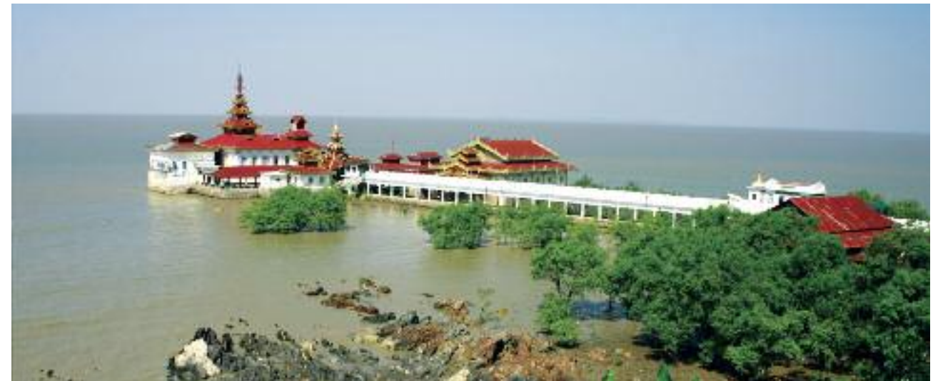
Kyaikkhami shrine, built on a rock outcrop in the sea. Its brick walls replaced a wooden structure destroyed by fire in the 1920s.
