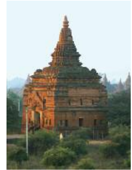
The sole surviving Hindu temple at Pagan is within the city walls. Dedicated to Vishnu, it may have been for royal rituals. Its outer brick wall and broad porch are missing, and the tower has been conjecturally restored.
