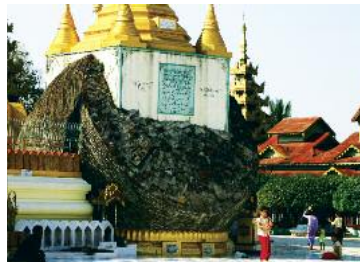
The massive chunk of brick that toppled in an earthquake in 1917 rests on the pagoda platform where it fell. The pagoda was rebuilt but collapsed again after a severe quake in 1930. It was not until the early 1950s that it was restored.
