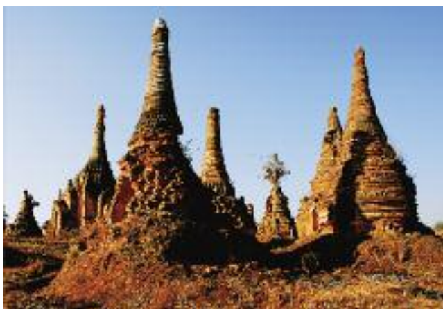
Ruinous stupas. When donors fail to fund ongoing maintenance, the weather and vegetation wreak havoc, hastened by damage caused by local treasure-seekers looking for precious objects. This cluster of mostly 19th century stupas surrounds the Indein Pagoda, Indein, Inle.
