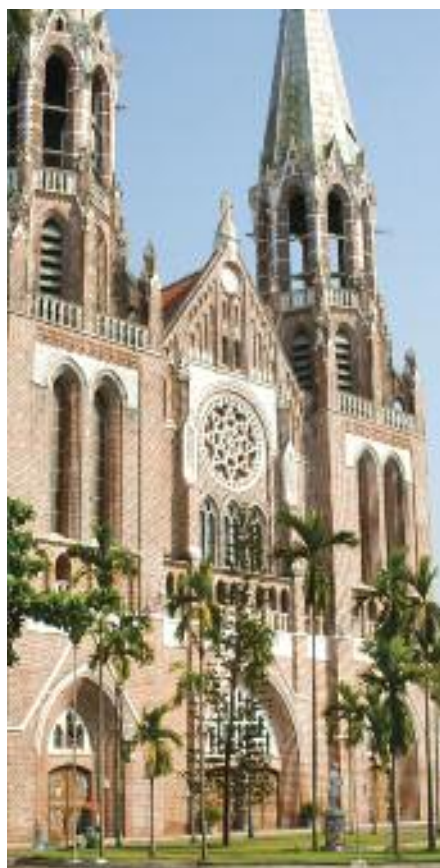
St. Mary's two heavy towers sank upon completion, wrenching the bond with the nave and nearly collapsing the cathedral.
