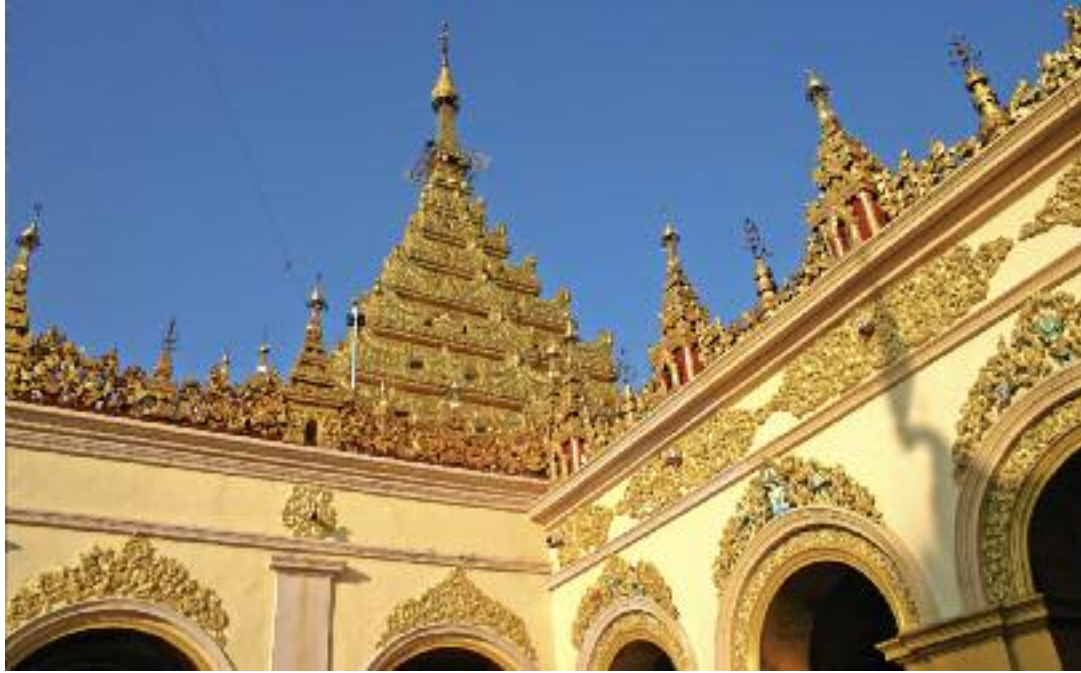
Hoynes Fox retained the existing inner sanctum, untouched by the 1884 fire, and capped it with a seven-storied tower that likely resembled the 18th century original. The arches are framed by painted plaster work affixed to wire armatures.
