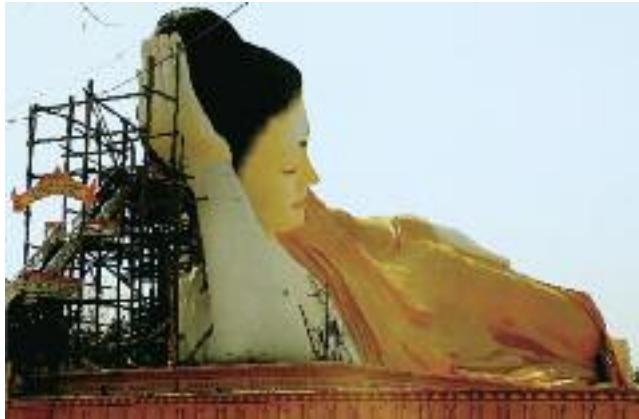
This new concrete reclining Buddha replaced a long brick mound that may have been a reclining Buddha. Demon tiles in the brick rubble suggest that it belongs to Dhammaceti's 15th century reign. It is located between the Kalyani Vihara and the Shwe-tha-lyaung reclining Buddha.
