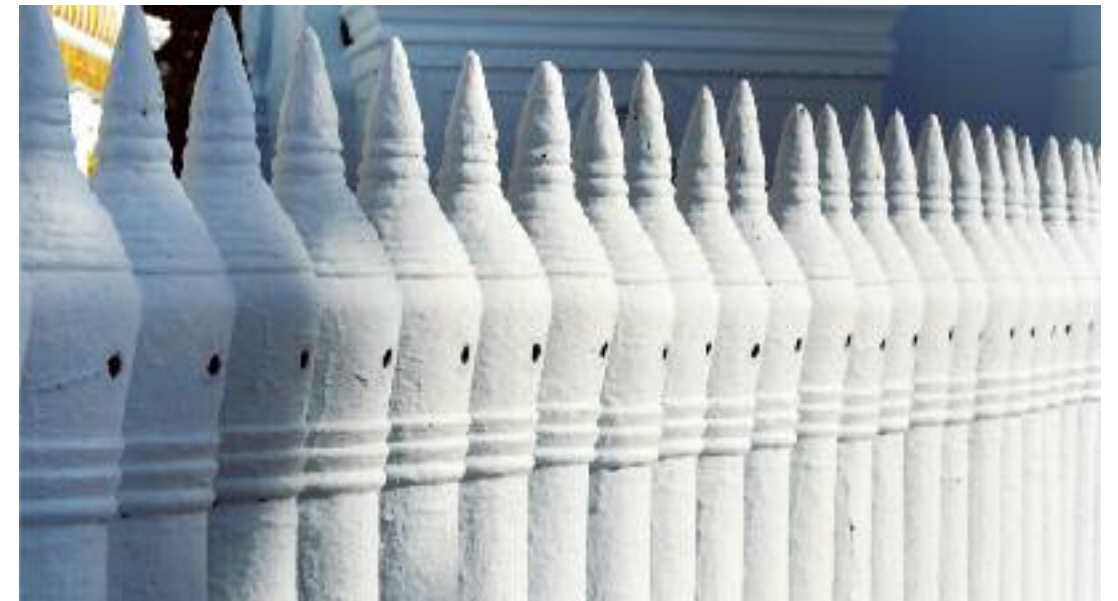
Lamps inside the tops of these tightly spaced stone posts give a special glow to the stupa's base. When these lamps were established is hard to say. Lamps also encircled the Shwedagon in Yangon, according to the pagoda's 15th century inscription.
