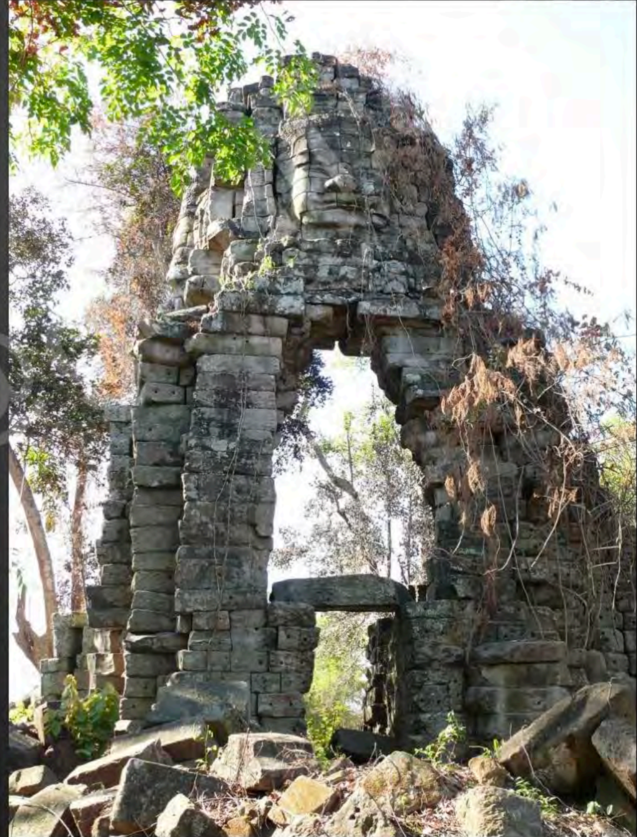
Current condition of the North side of the face tower of the satellite-temple IV (March 2010)
