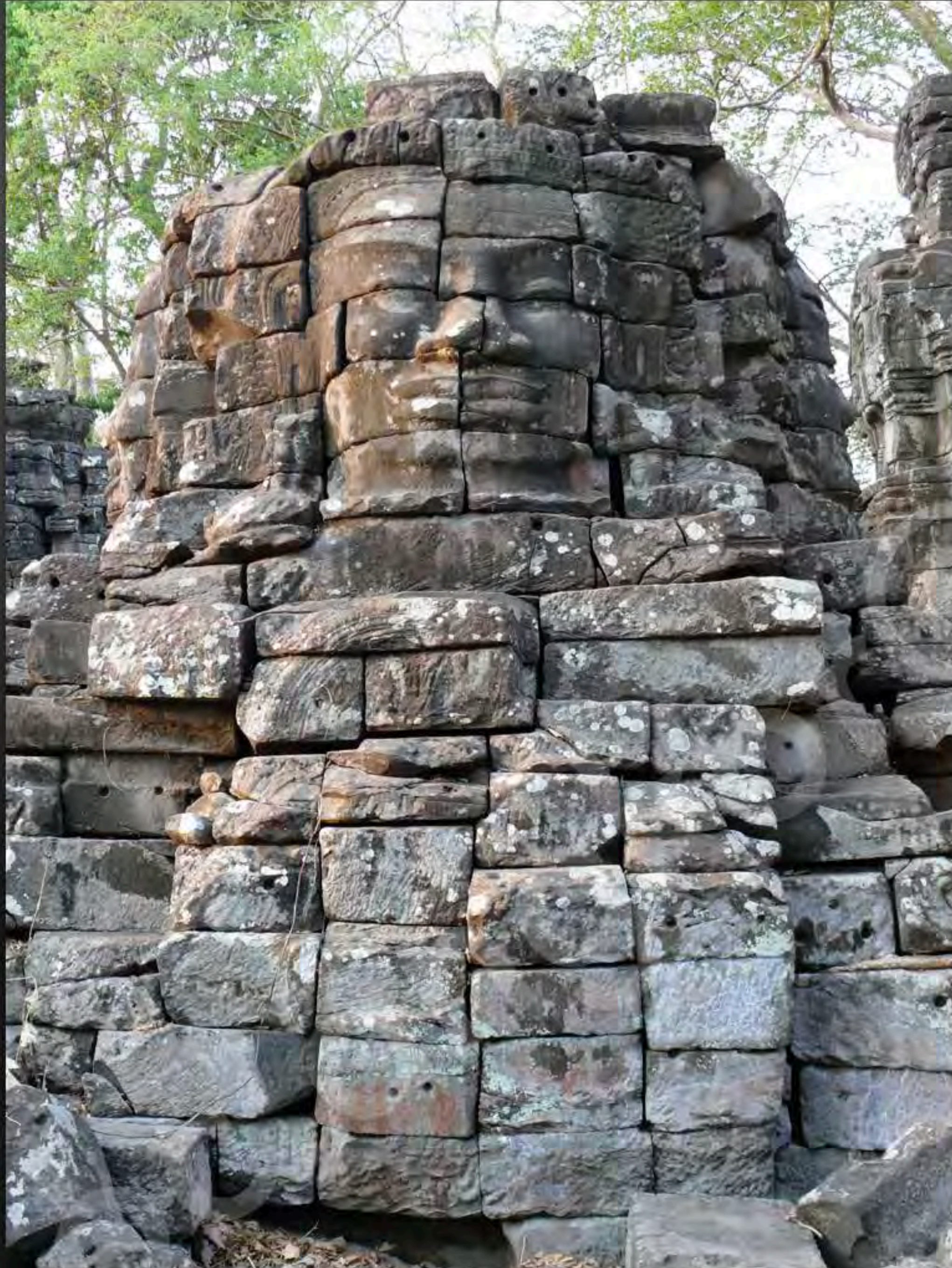
Current condition of the South side of tower 15 of the 1 st enclosure (March 2007)
