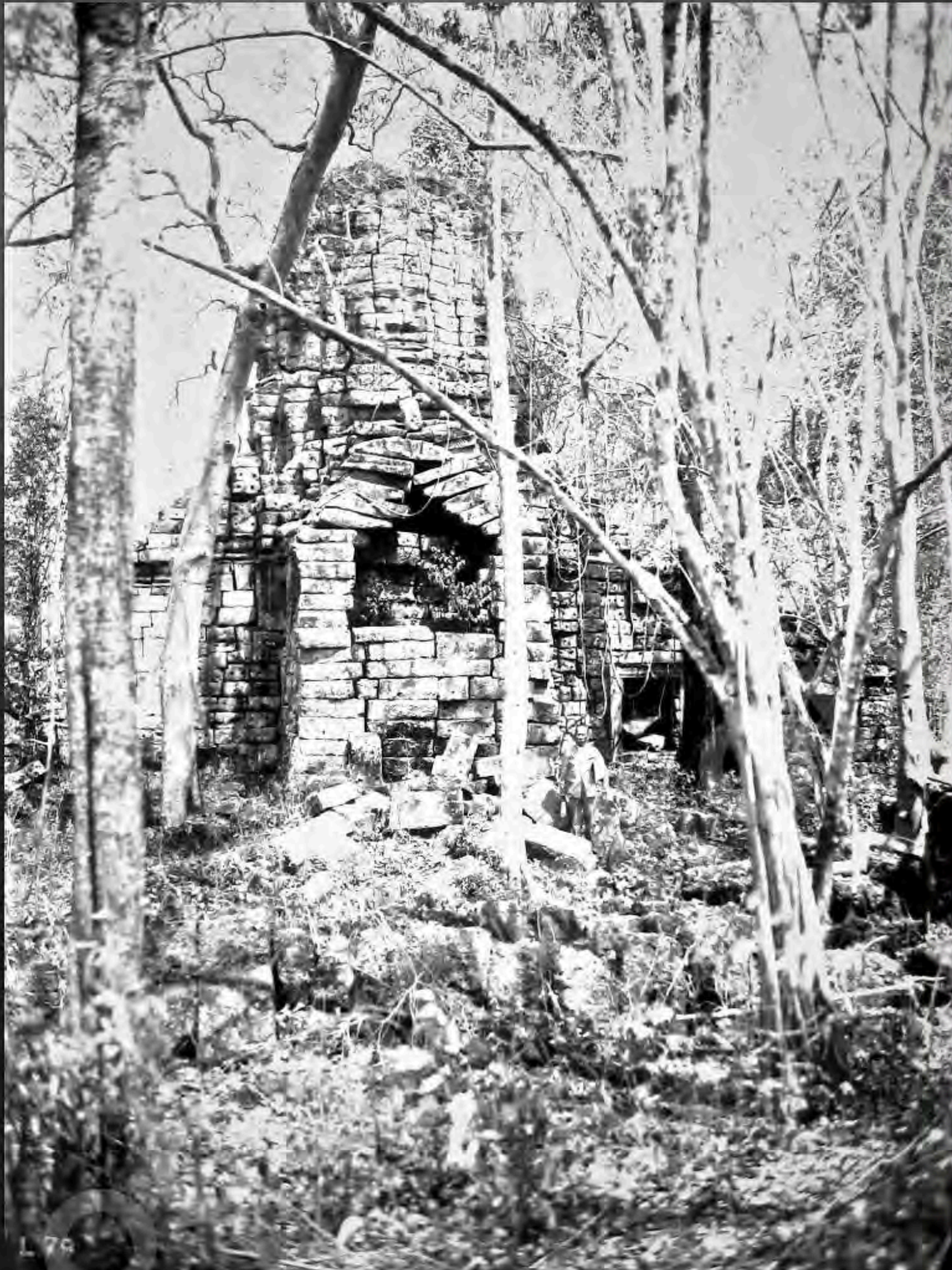
Condition of the South side of the face tower of the satellite-temple V in February 1932 (G. Groslier - © MCFA - 128.5)
