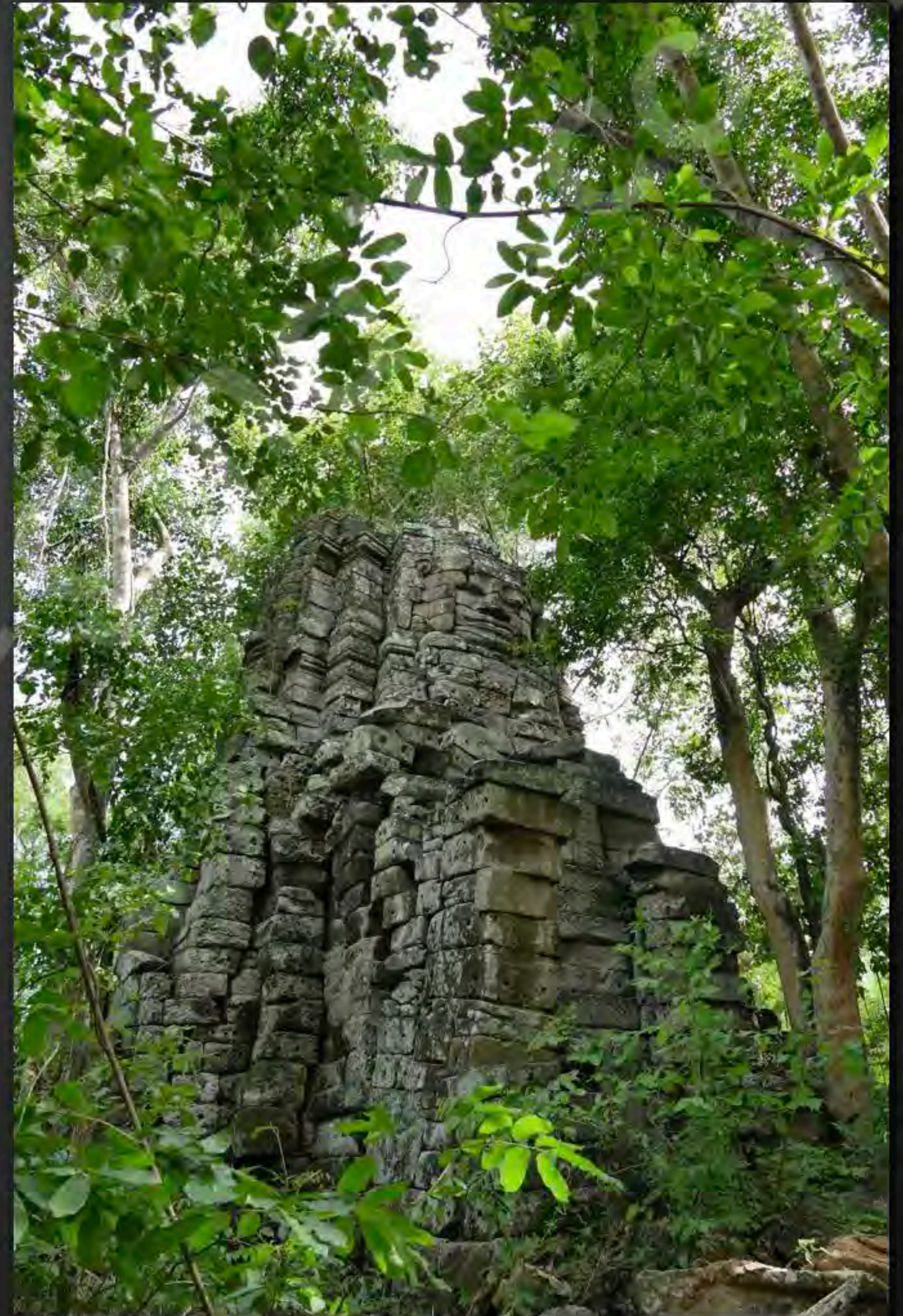
Current condition of the North side of the face tower of the satellite-temple III (July 2015)
