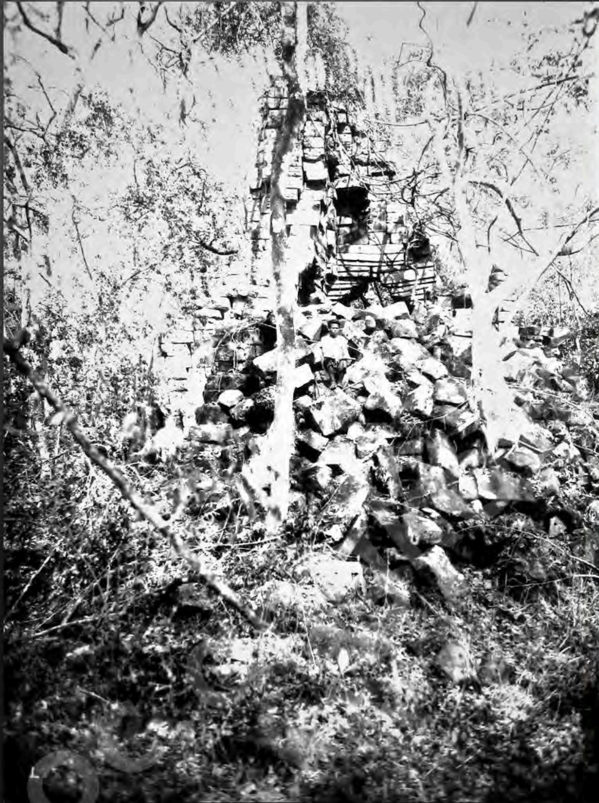
Condition of the West side of the face tower of the satellite-temple III in February 1932 (G. Groslier - © MCFA - 128.3)
