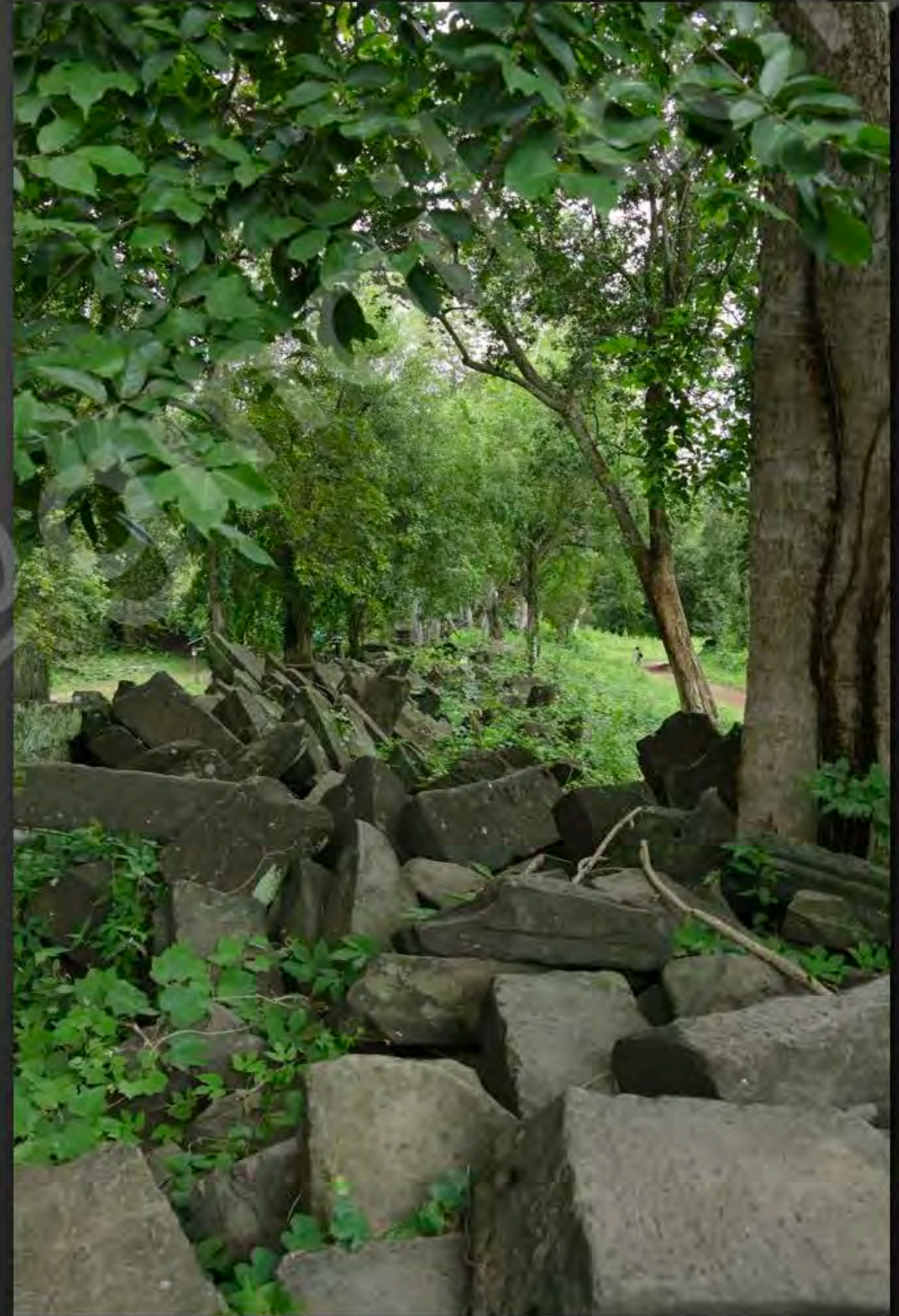
Current condition of the East wing of the Northern gallery View from East to West (September 2015)
