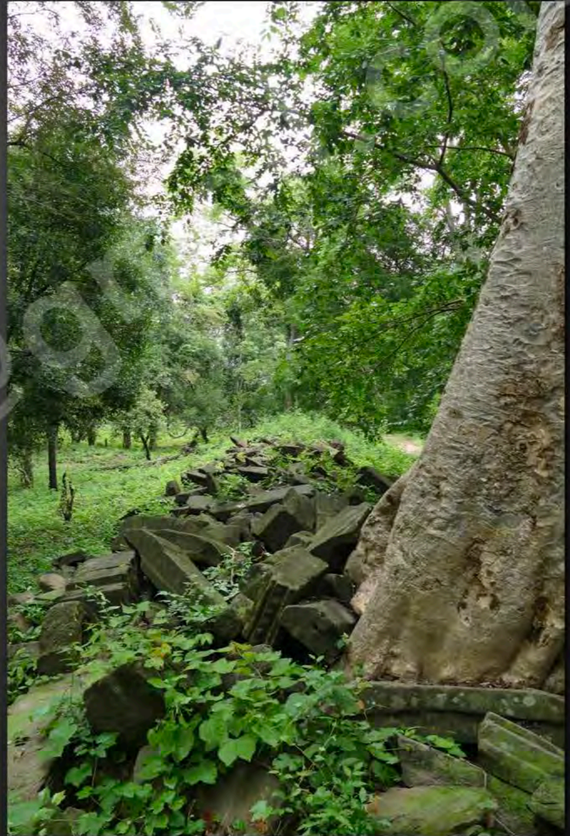
Current condition of the West wing of the Northern gallery View from East to West (September 2015)
