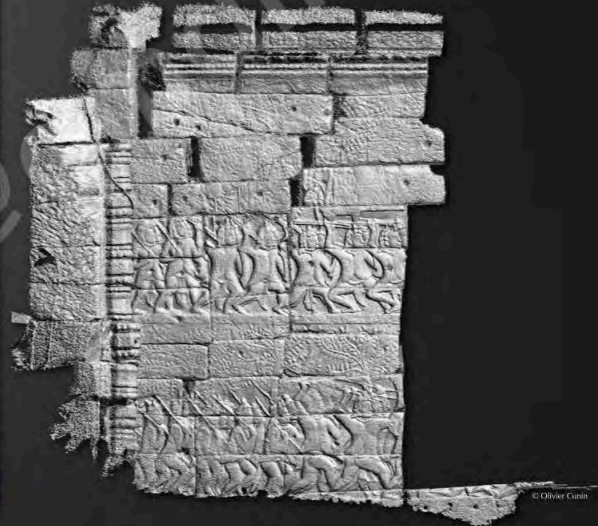
3D scanning by photogrammetry of the current condition of the East end of the West wing of the Northern gallery
