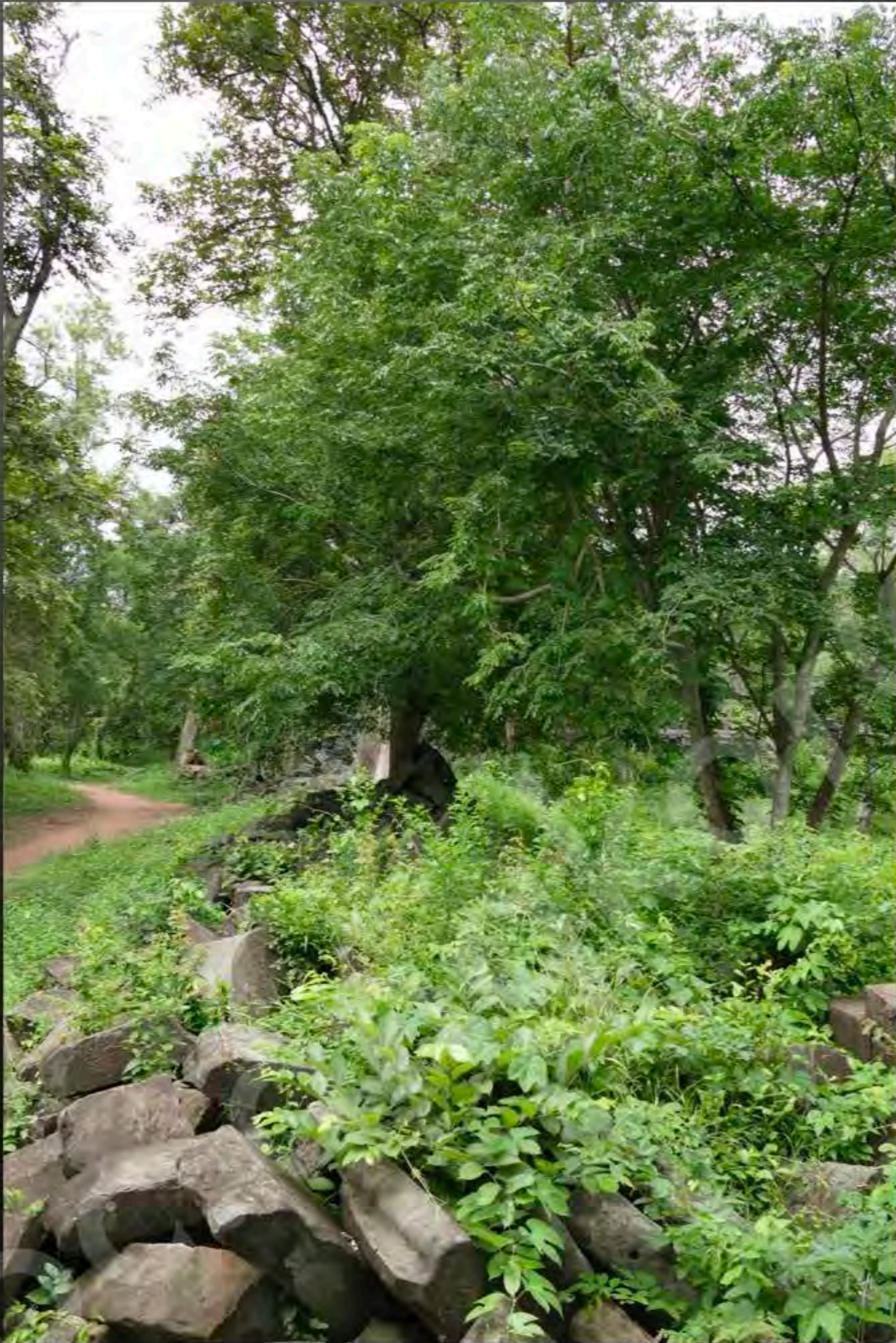
Current condition of the West wing of the Northern gallery View from West to East (September 2015)
