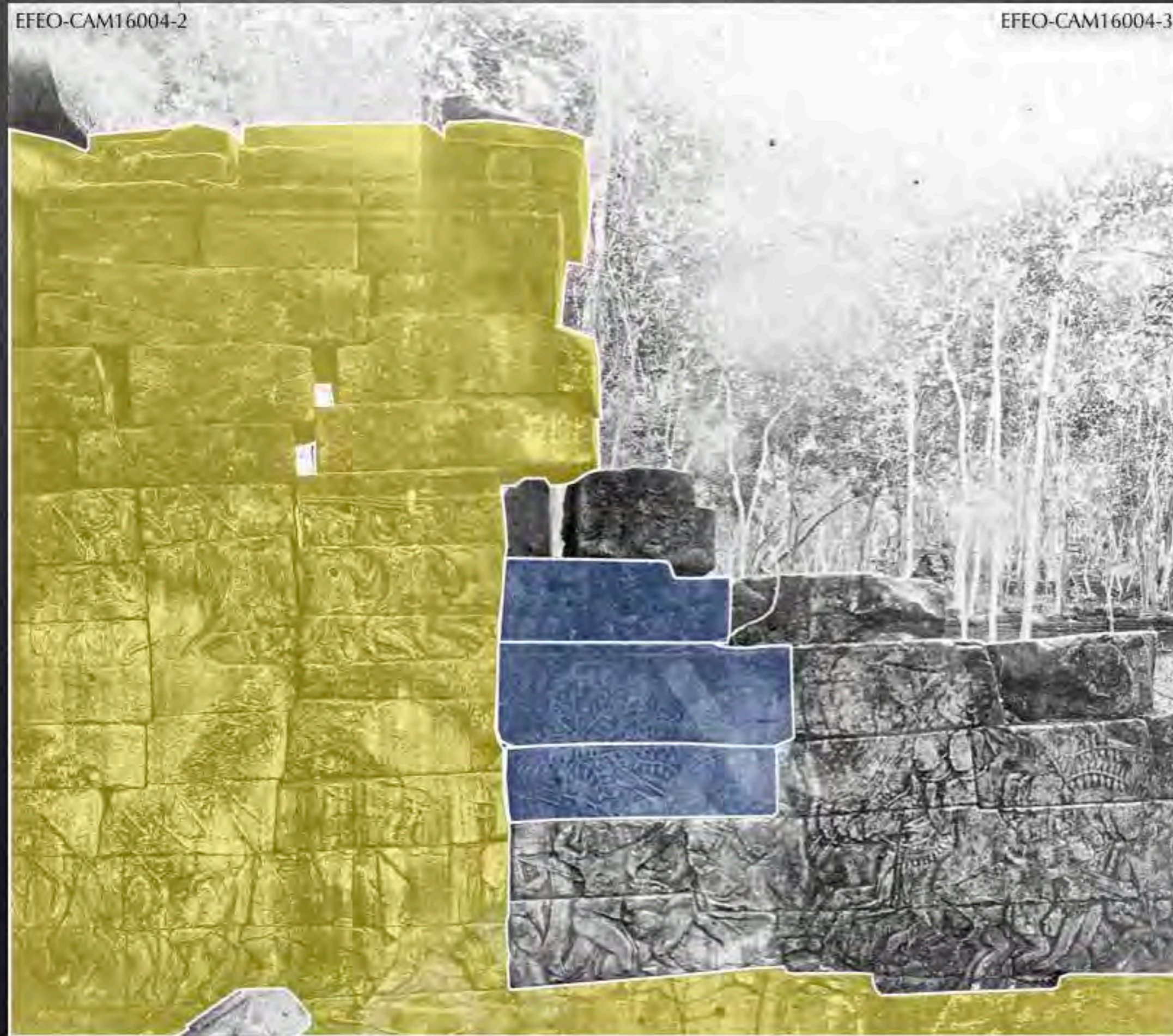
Condition in 1909 of the East end of the West wing of the Northern gallery (Photomontage of the photos of General de Beylié from the photos archives of the EFE0)
