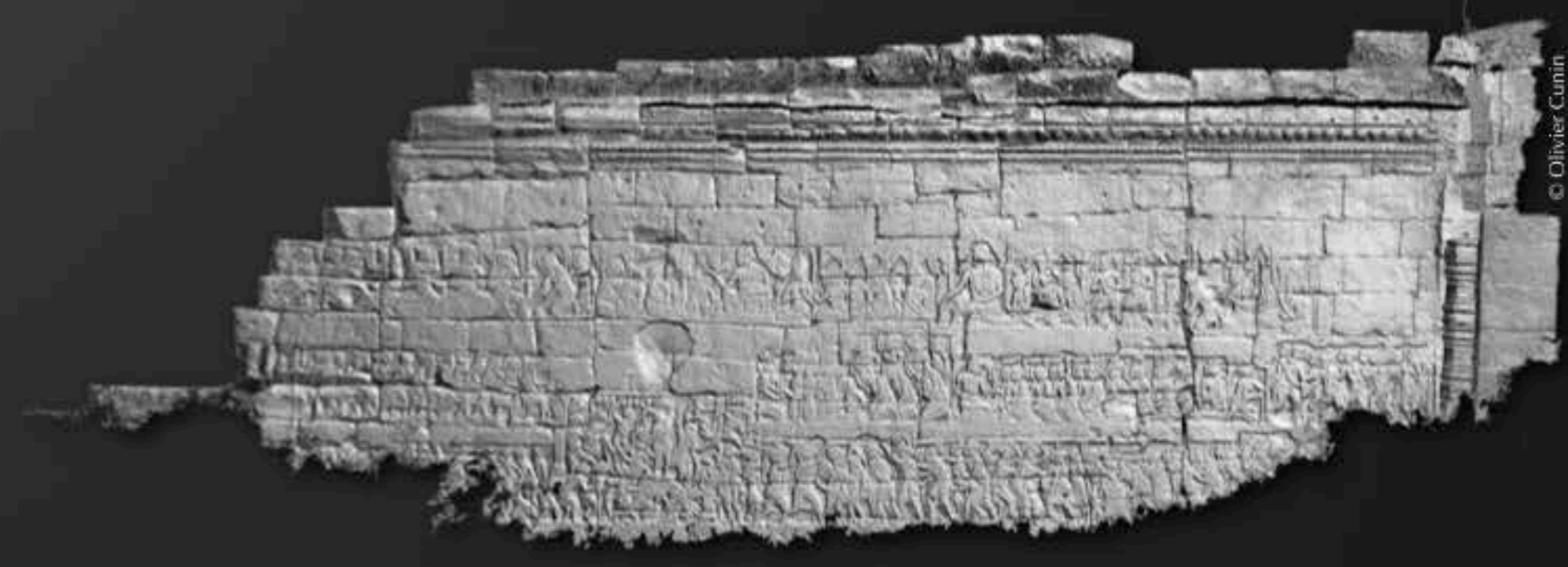
3D scanning by photogrammetry of the current condition of the South end of South wing of the Western gallery
