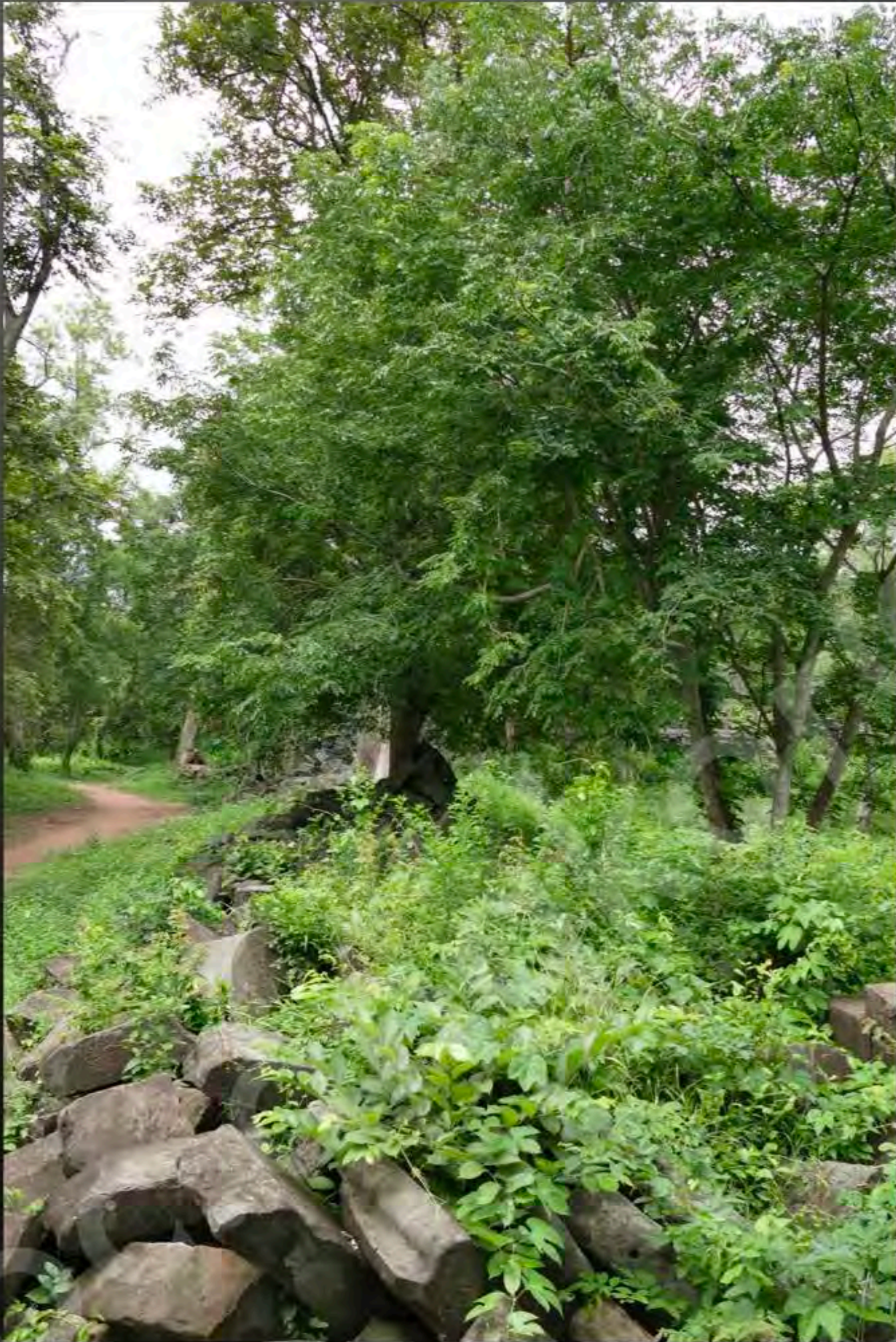
Current condition of the South wing of the Western gallery View from South to North (September 2015)
