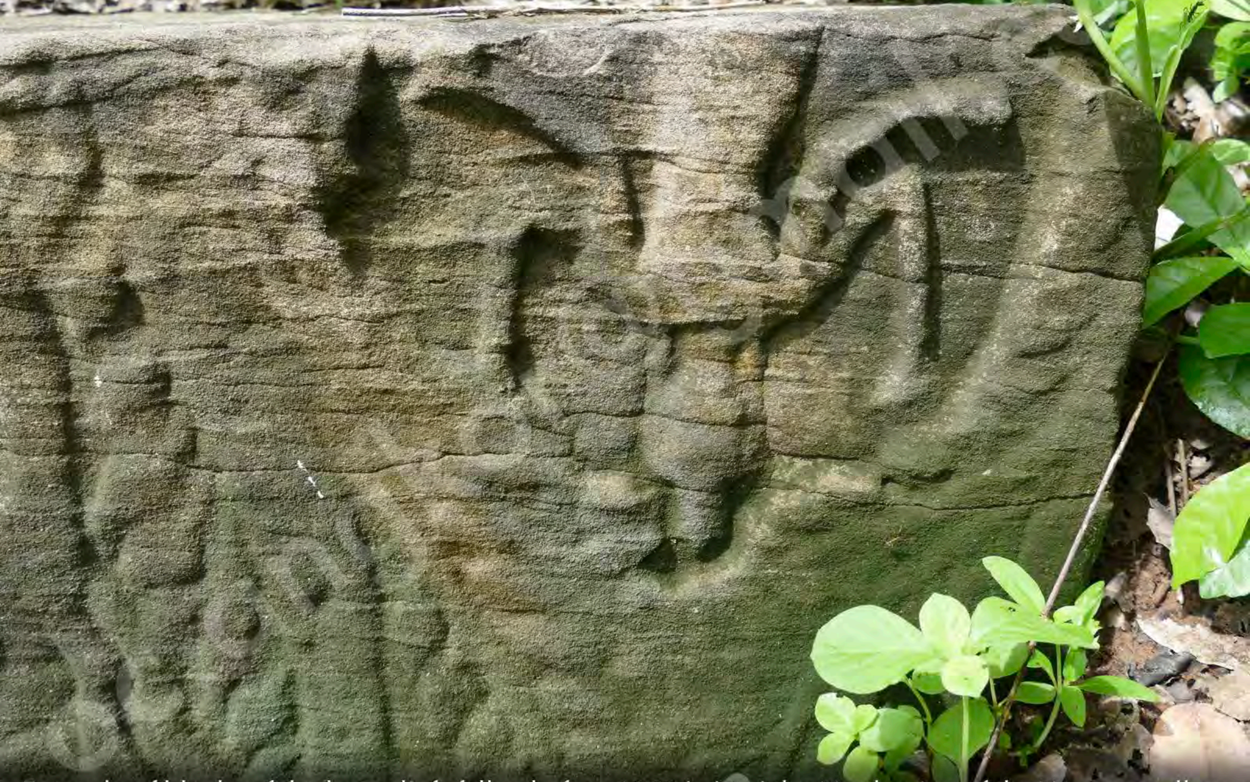
Example of blocks of the bas-reliefs fallen before 1909 behind the North wing of the Western gallery
