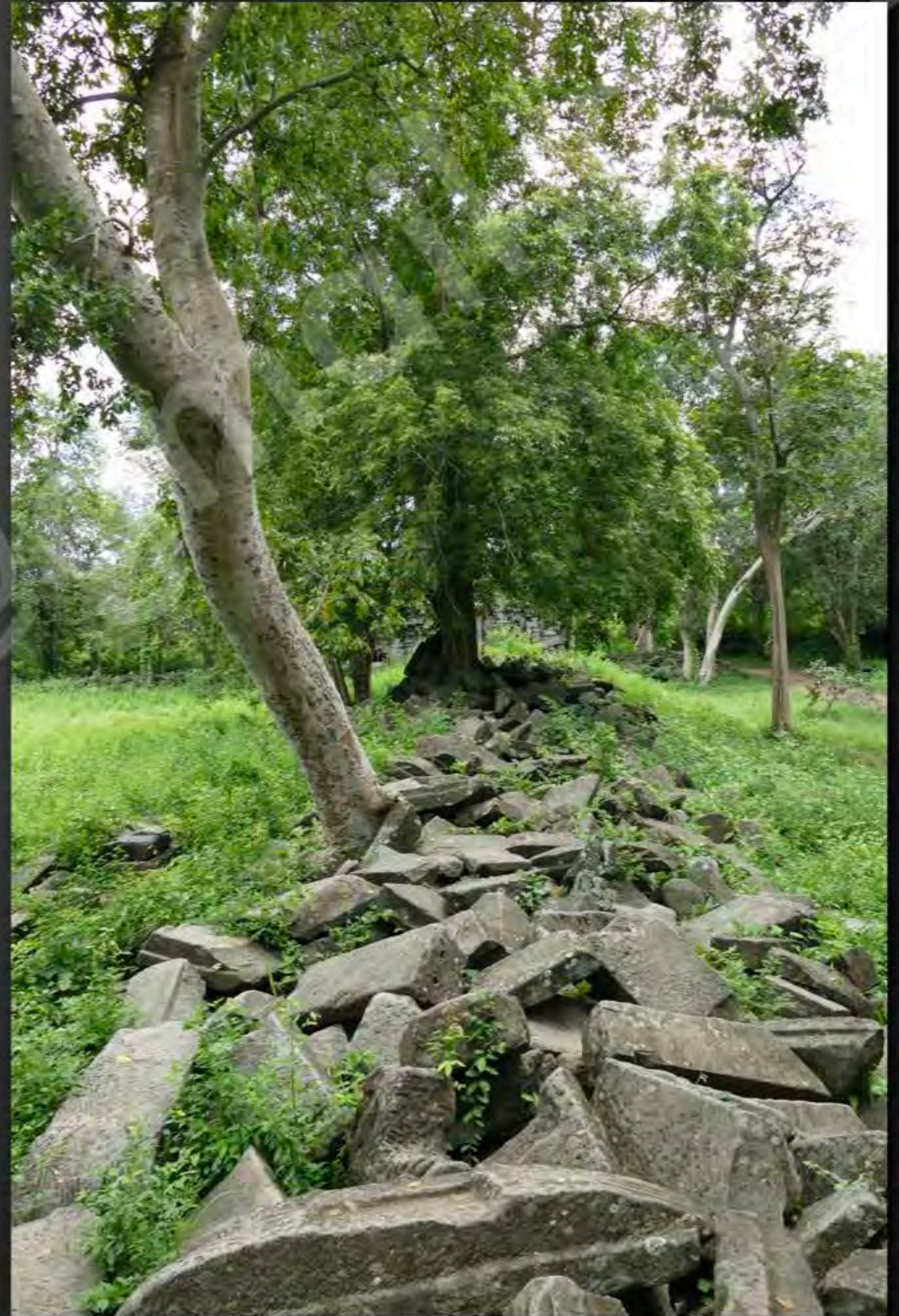
Current condition of the South wing of the Western gallery View from North to South (September 2015)
