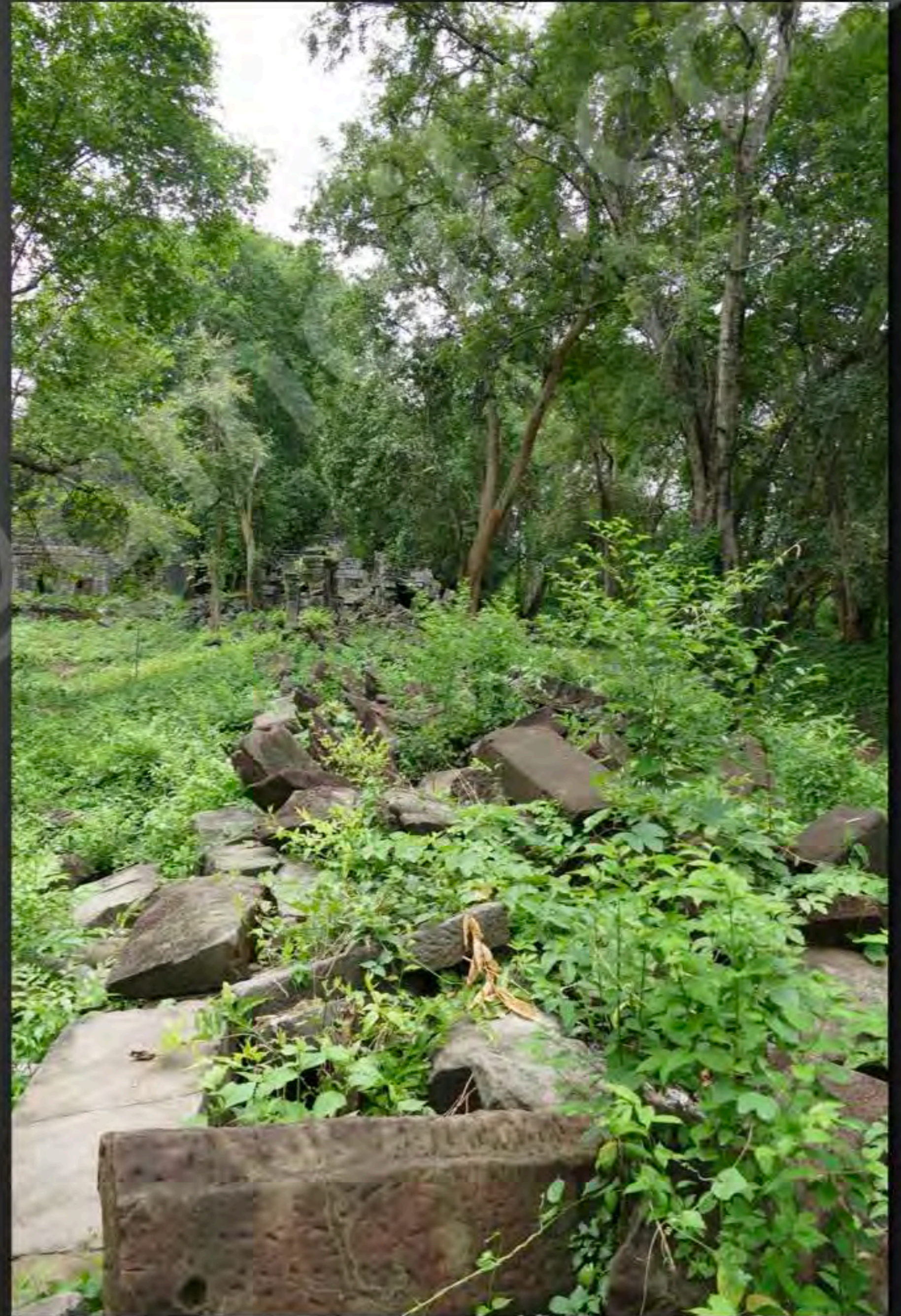
Current condition of the North wing of the Western gallery View from North to South (September 2015)
