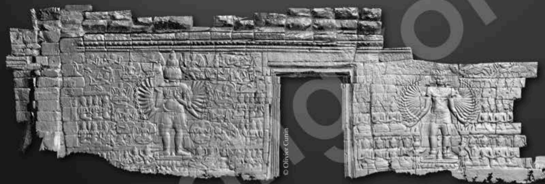
3D scanning by photogrammetry of the current condition of the North end of South wing of the Western gallery
