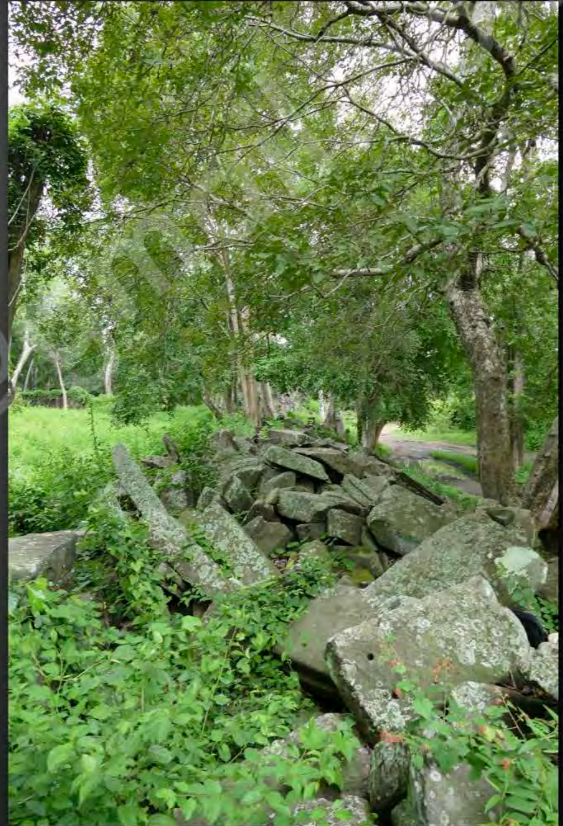
Current condition of the West wing of the Southern gallery View from West to East (September 2015)
