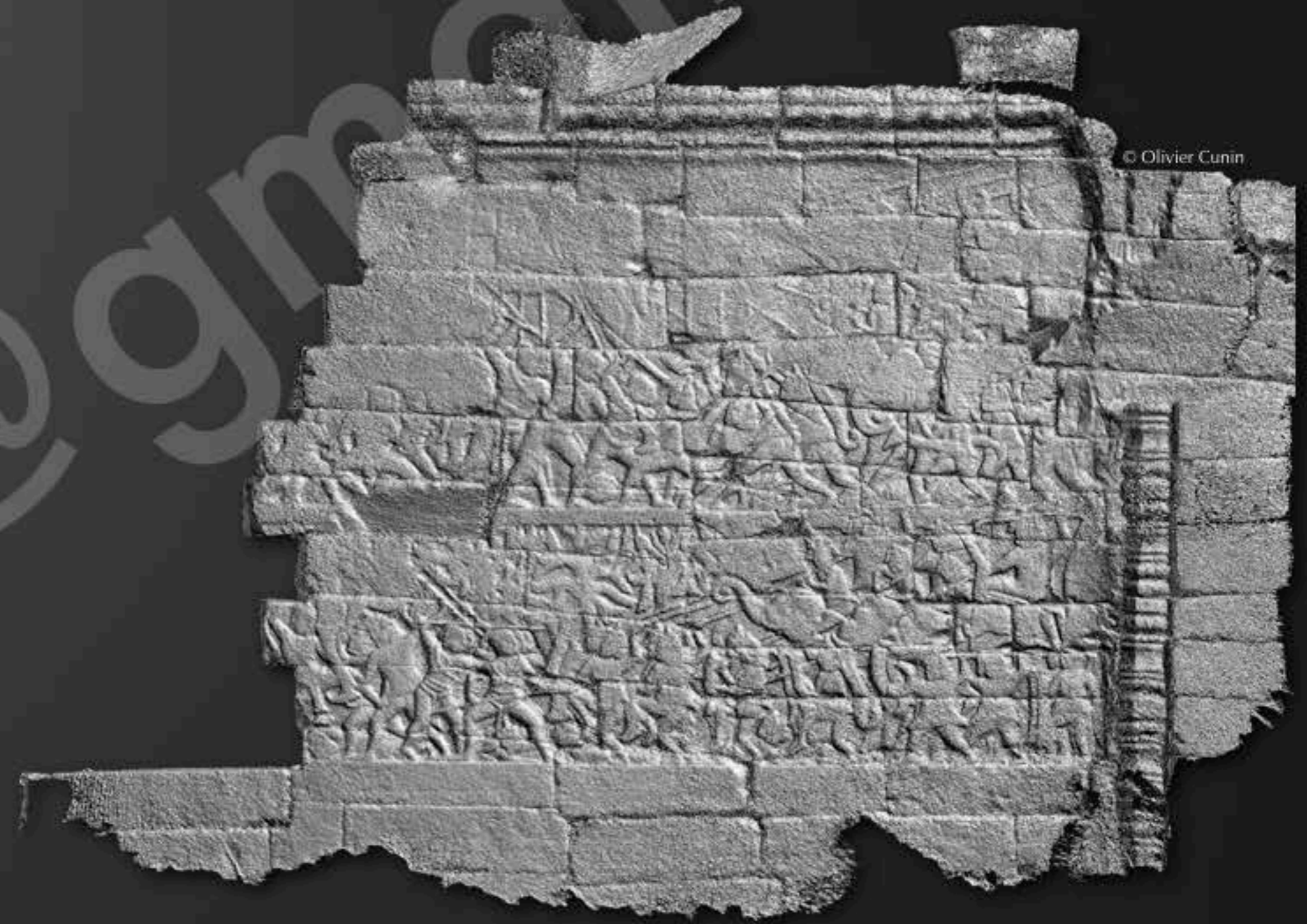
3D scanning by photogrammetry of the current condition of the East end of the East wing of the Southern gallery
