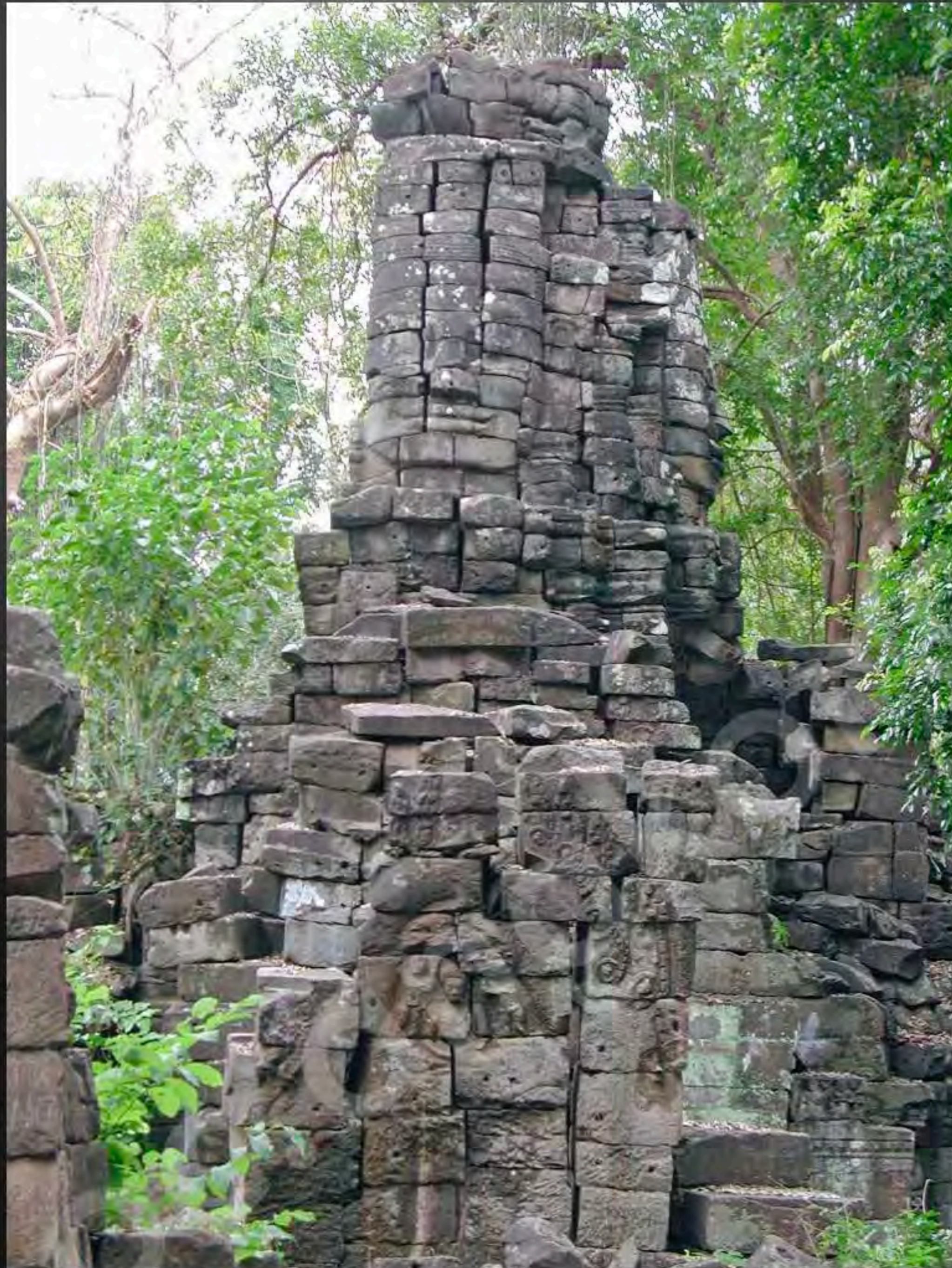
North face of tower 73 of the West group of the 2 nd enclosure in December 2002
