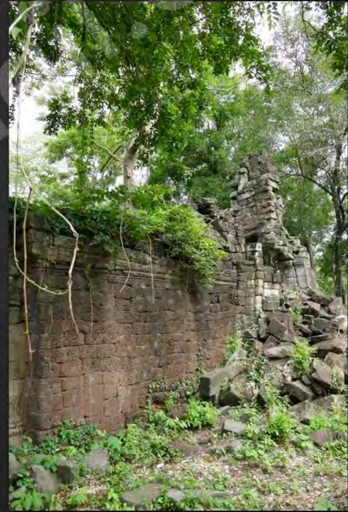
Current condition of the tower 70 of the Western of the 2 nd enclosure view from the Northwest (Septembre 2015)
