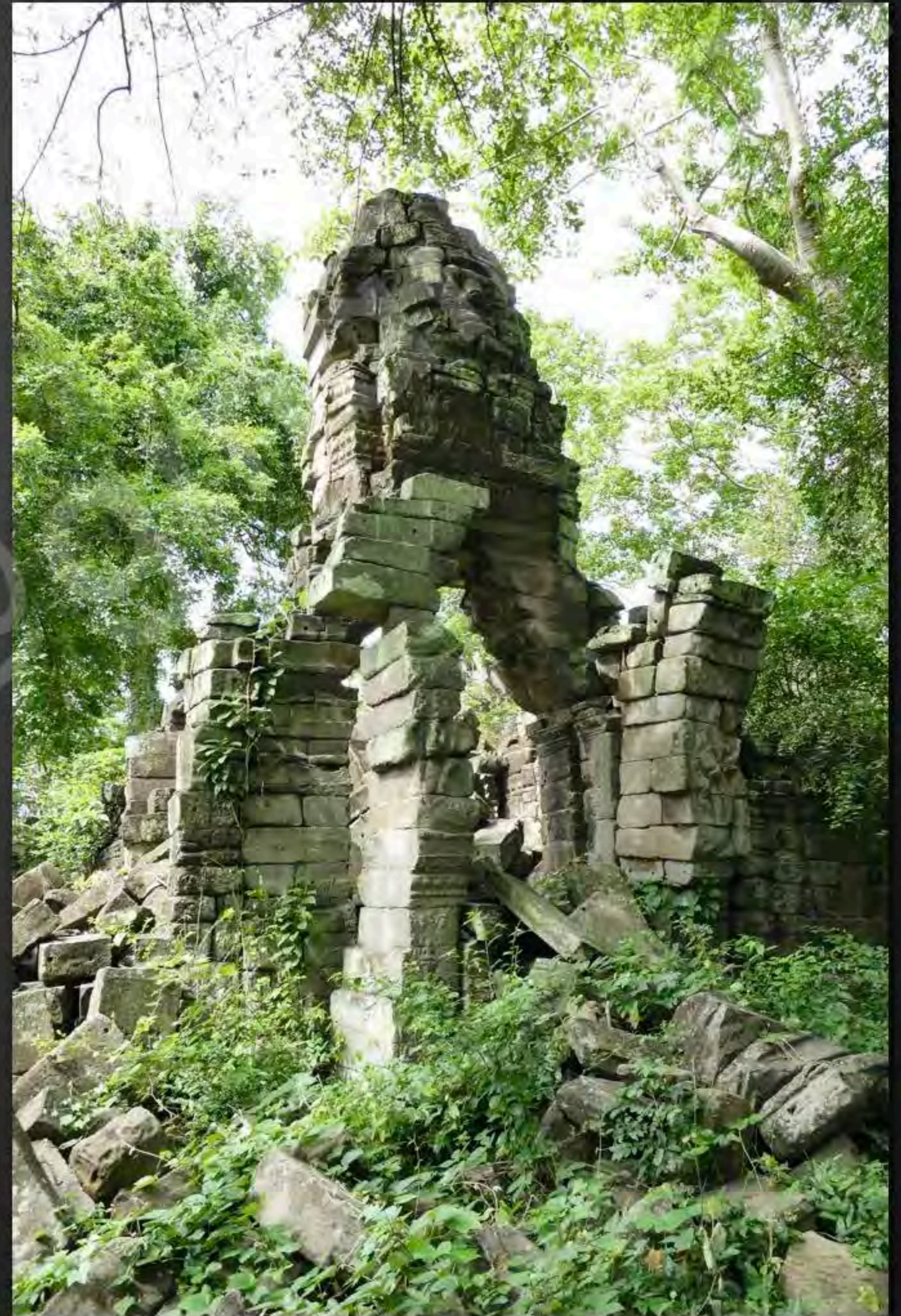
Current condition of the South side of tower 70 of the Western of the 2 nd enclosure (September 2015)
