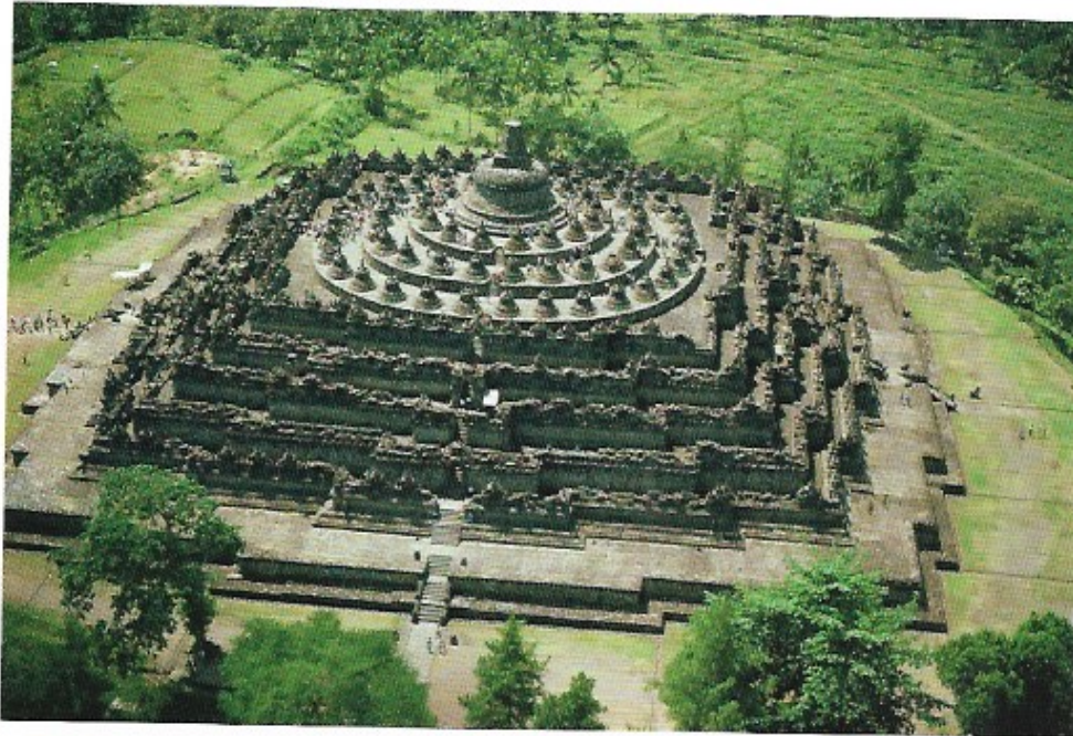
Fig 54.9 Aerial view of Candi Borobudur, Magelang, Central Java, Indonesia (c. 780–830). This stepped temple complex from the Shailendra dynasty has five square terraces on which sit three circular terraces and a central stupa. The life-size Buddha figures placed in the external niches are the monument's key architectural feature. The small stupas on the circular terraces also enclose a life-size Buddha figure.
