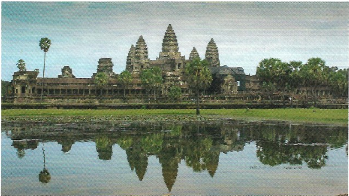
Fig 54.14 Angkor Wat, Angkor Archaeological Park (1113–50). This celebrated temple complex was erected by King Suryavarman II. Its central tower, known as bakan , is seen here along with the four other flanking towers. The richly carved, corn-cob-like superstructure of these towers, or prangs , remained the central architectural feature of Khmer Empire temples throughout the Angkor period.
