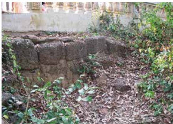
Ph. 36 Basement of Vihear, laterite blocks
