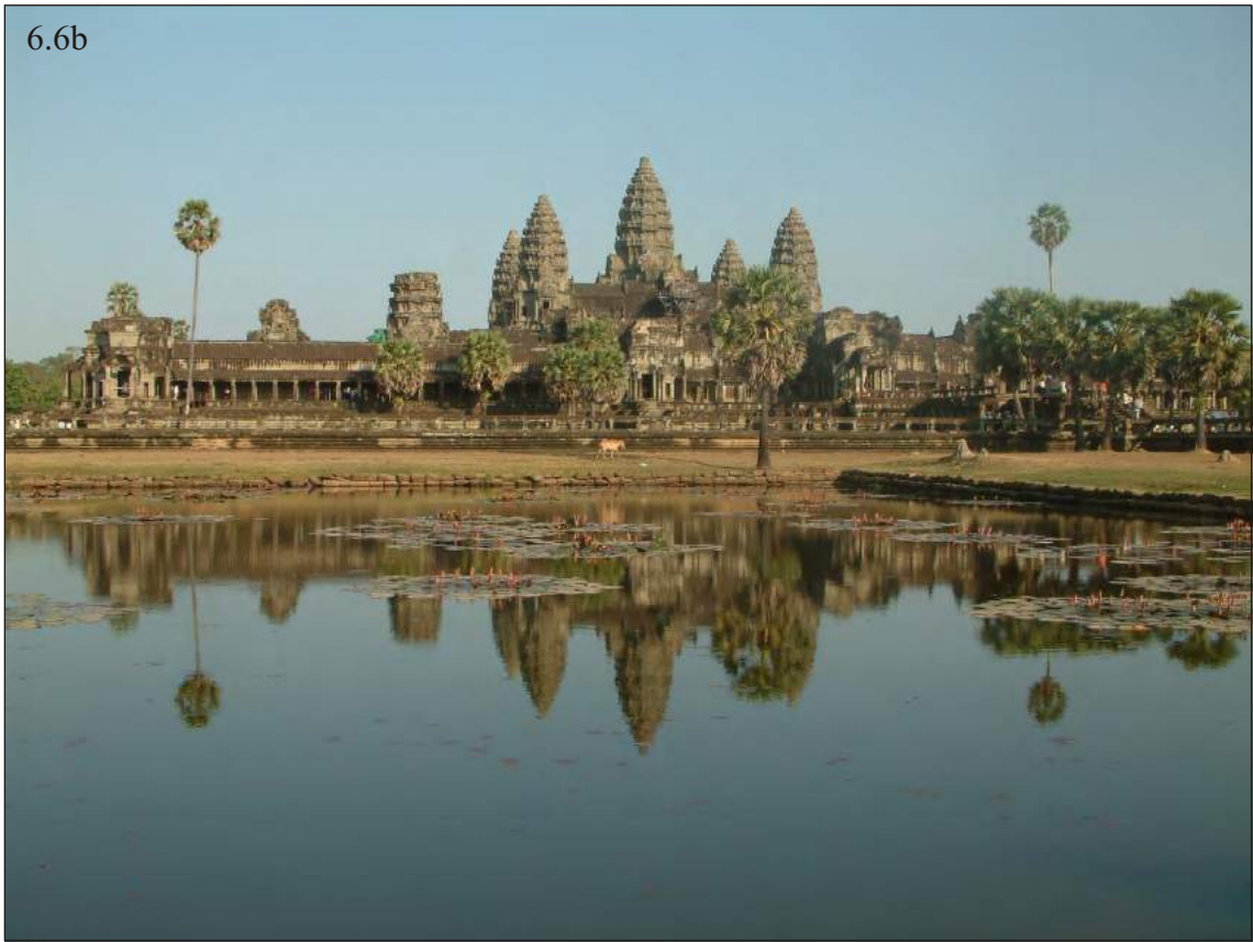
Figure 6.ba-b Variation in number of towers (a) single tower at Prasat Neang Khmau, Koh Ker and (b) quincunx arrangement of Angkor Wat
