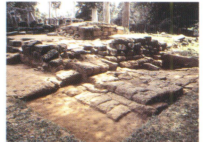
Figure 8. Southeast Platform C10, CU03 and CU04, see from the south.
