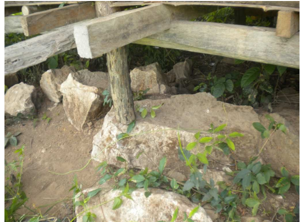
Fig. 24 - Jar used as foundation for pillars, Site 38. © Lia Genovese (June 2011)
