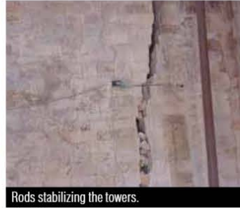
Rods stabilizing the towers.
