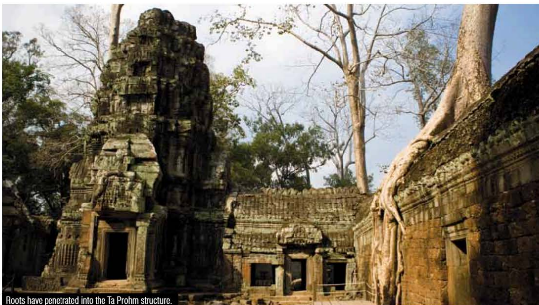
Roots have penetrated into the Ta Prohm structure.
