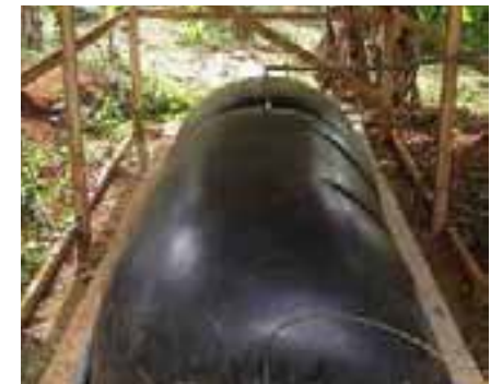
▲ A biogas digester. The family adds animal manure to the bag, which then breaks down to produce gas which can be used for cooking.
