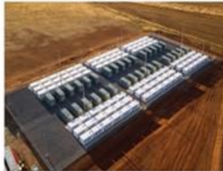
Figure 5: Typical Battery Storage Facility
