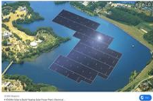
Figure 4: Typical floating solar system (14)
