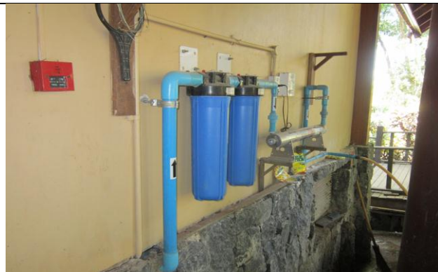
Water purification system attached to the kitchen
