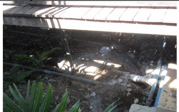
Bio-tank installed under bungalow
