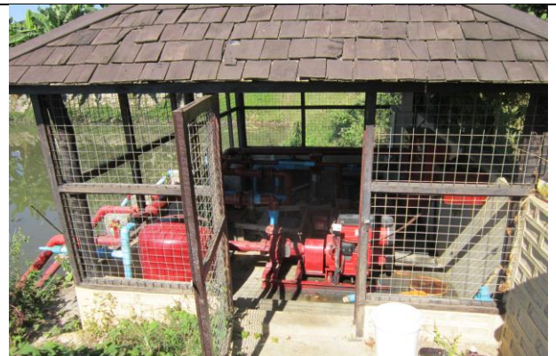
Emergency water pump
