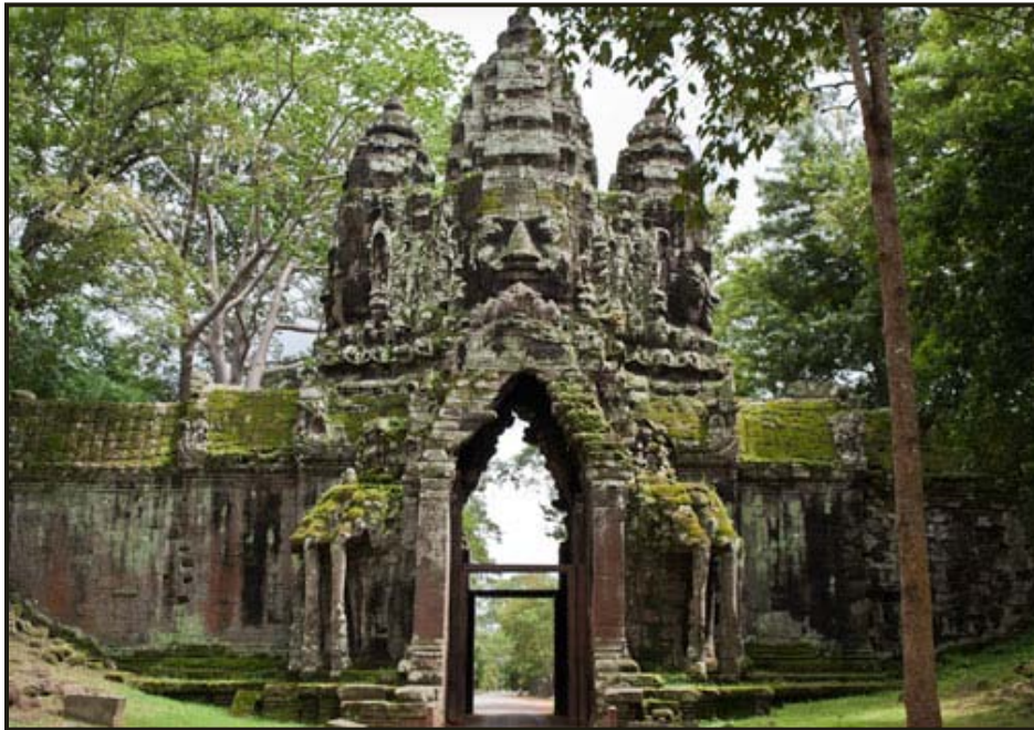
North gate of Angkor Thom, note the paired 3-headed elephants and missing pediments with the facades, thus exposing the roofing's frame into the king's giant faces.
